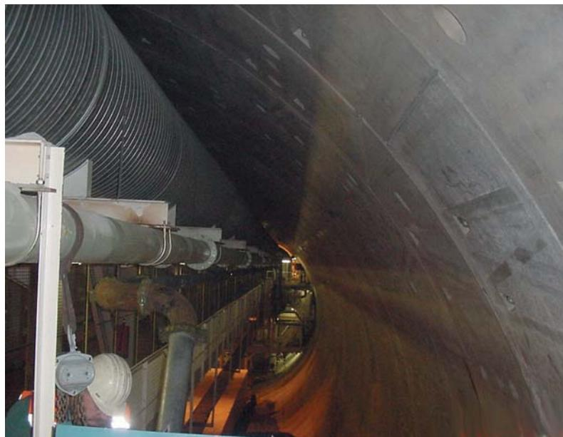
14.9 m in diameter is one of the biggest drills in the world, that is used to build the largest railway tunnel in the Netherlands. In this application KLINGER Ballostar ball valves are applied for Betonit injection and for the transport of mud. Our products meet the highest requested requirements under difficult conditions.
