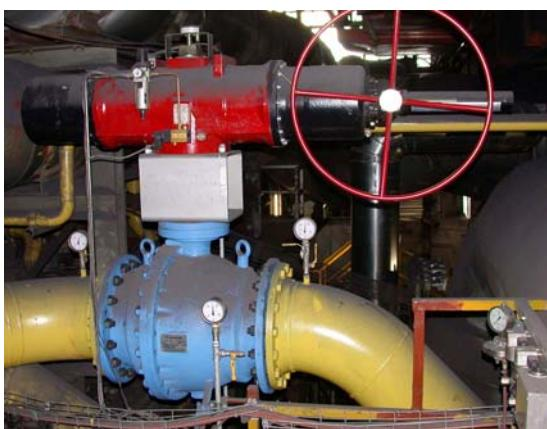
KHI DN 400 equipped with pneumatic actuator
